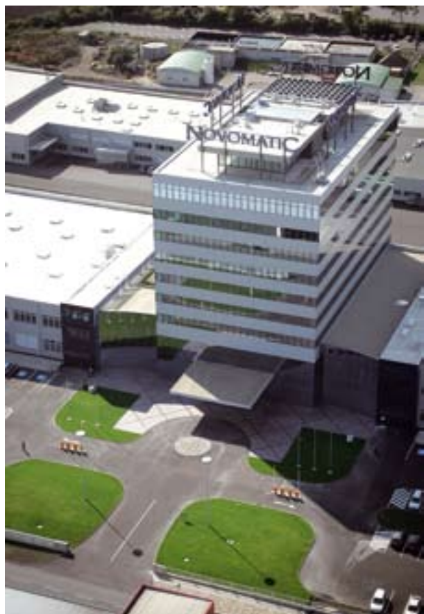
Novomatic Headquarters in Gumpoldskirchen.
